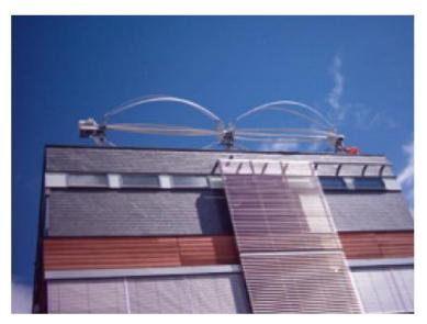
Figure 2.15: Windwall turbine in the Hague
